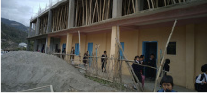
An AVP School building under construction in Namsai, Arunachal Pradesh
