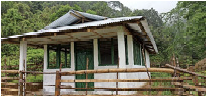
A Community Activity Center (CAC) building in a village in Arunachal Pradesh
