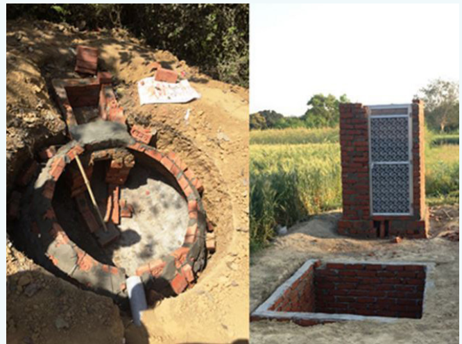
A Bio-Toilet under construction
